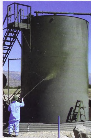
Apply the base coat.
